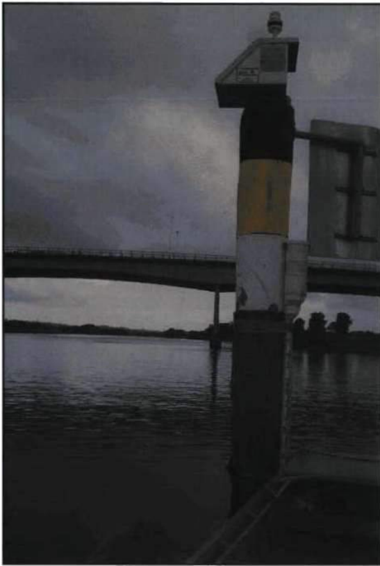
■ Figure 2-3 Tide gauge at Silverwater Bridge
